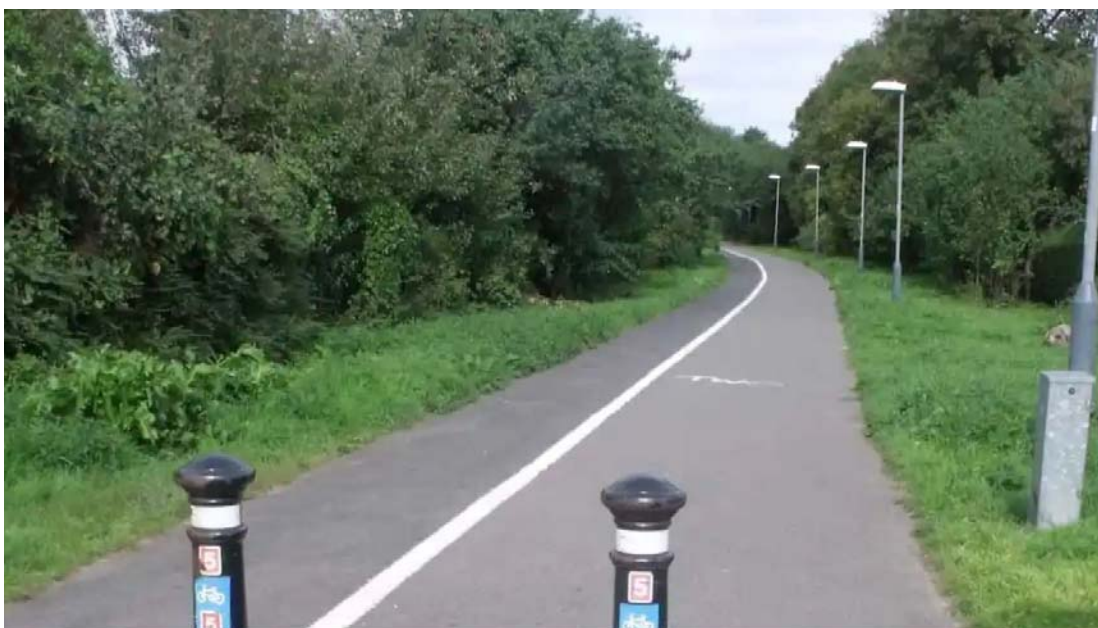
National Cycle Network Route 5 in Warwick, which is similar to the Europa Avenue proposal
